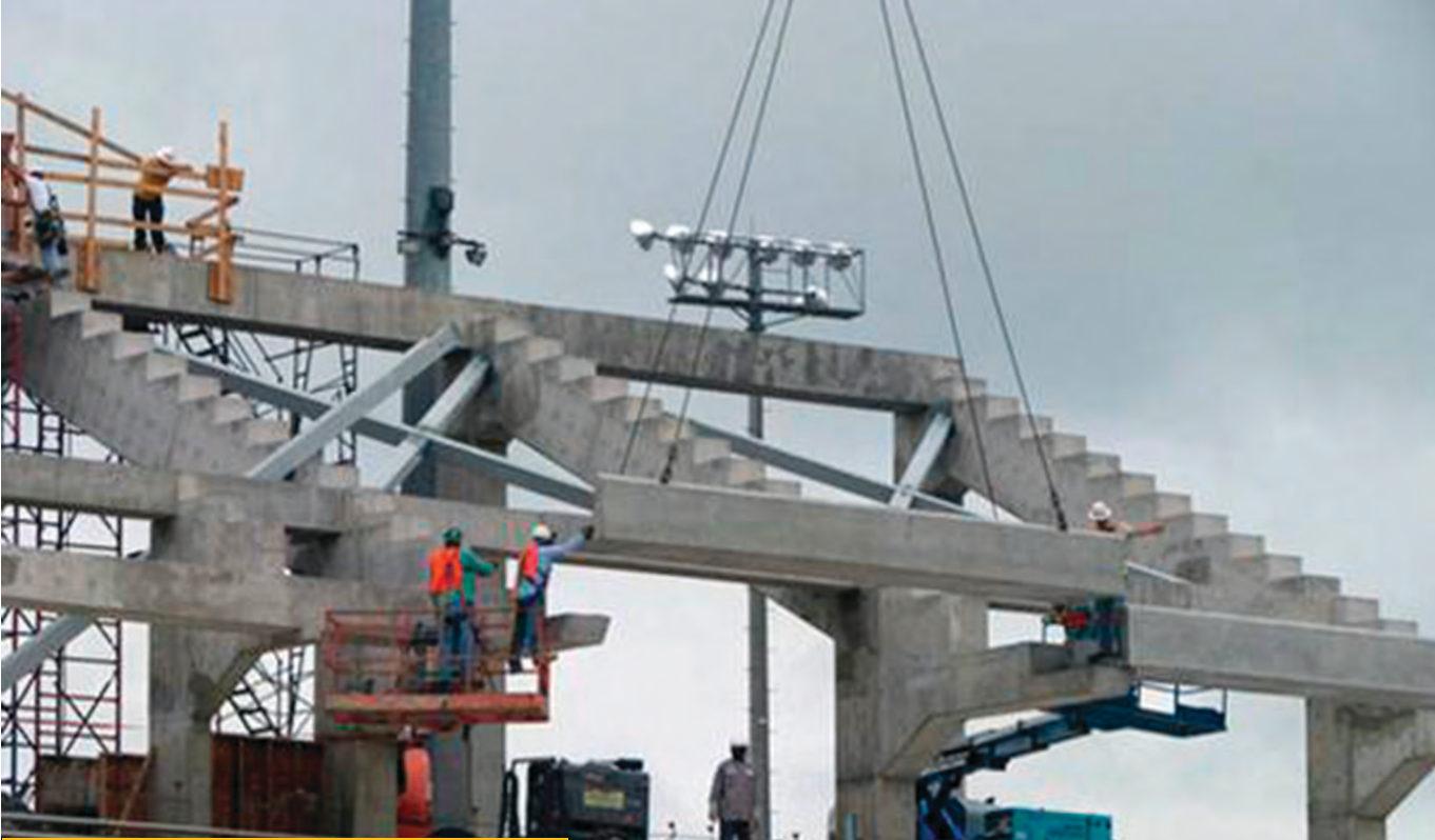
PRECAST RACKER BEAMS
