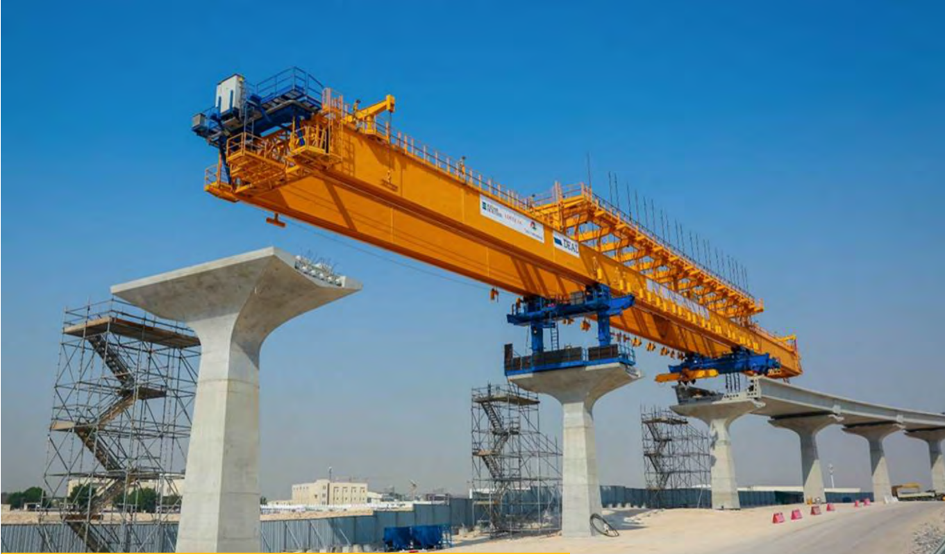
QATAR RAIL RED LINE ELEVATED PROJECT
