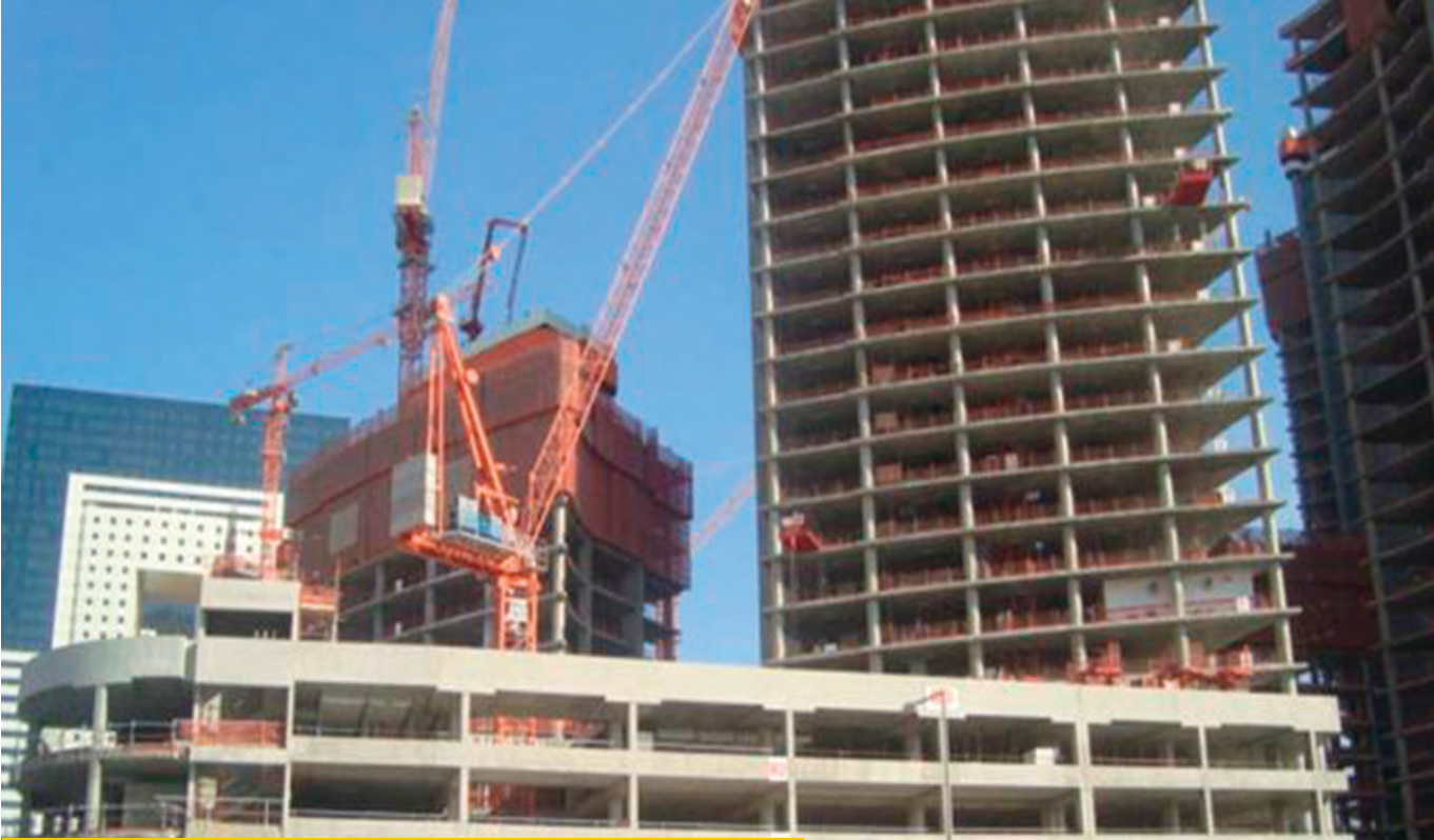
BARWA FINANCIAL DISTRICT-CAR PARK
