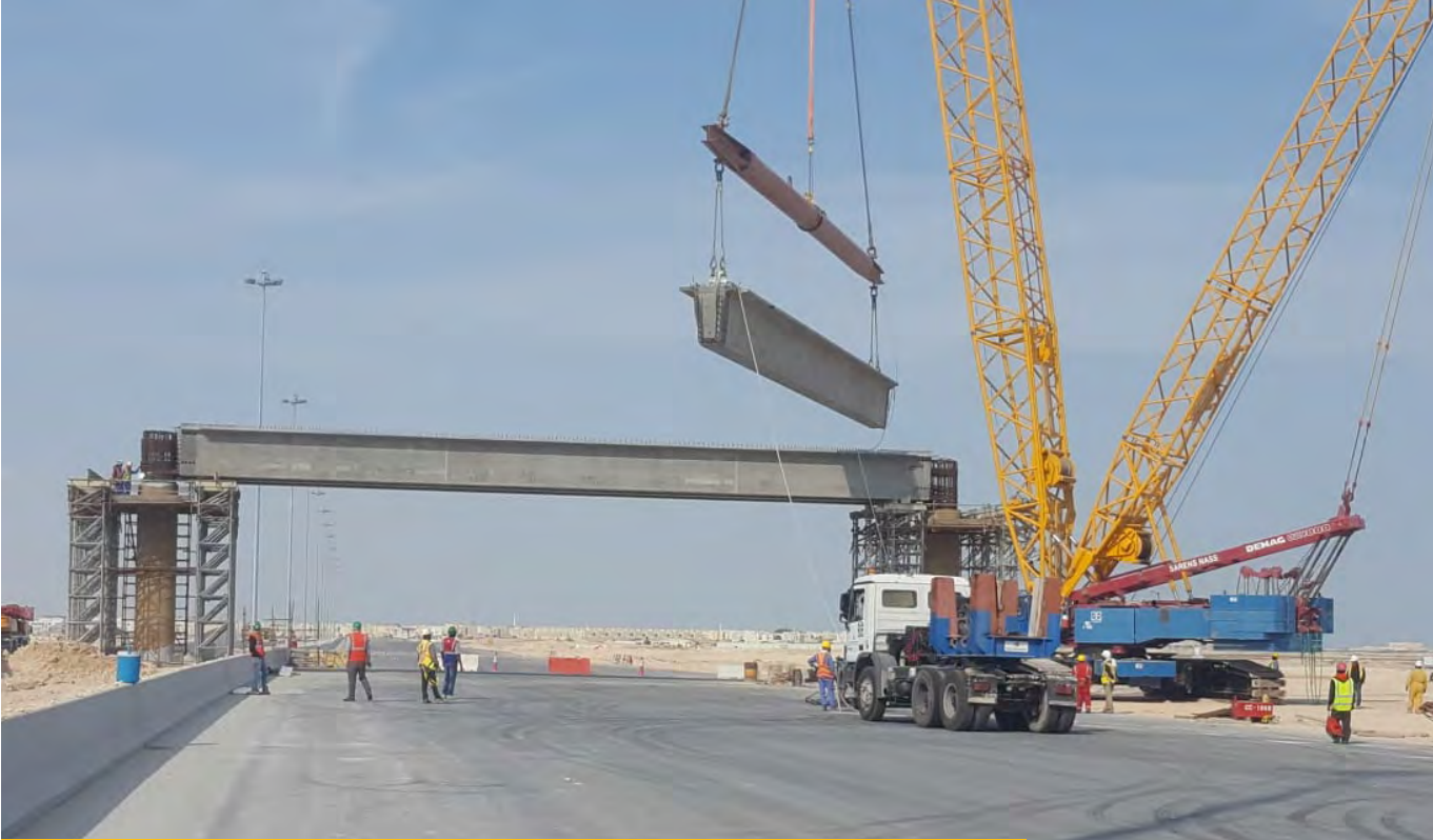
ERECTION OF GIRDERS AT E RING ROAD PROJECT
